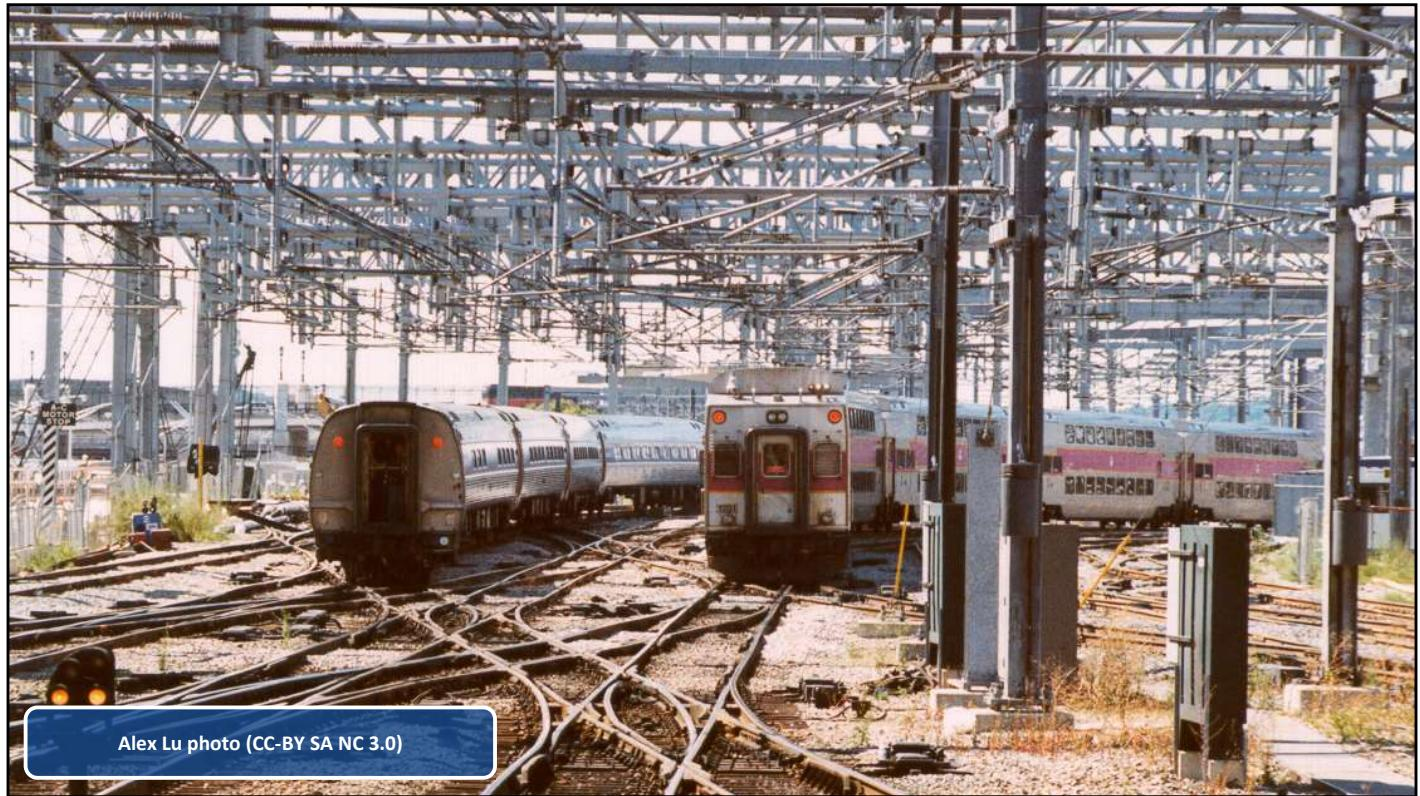
Most rail professionals have some experience with routing trains around a track obstruction, making moves using appropriate signals, crossovers, and tracks. Isolating a segment of overhead catenary is similar in concept, but outages must provide electrical paths to deliver power outside the de-energized area, keep crossovers and drawbridges energized whenever possible, and ensure that the power supply doesn't become "unbalanced".
